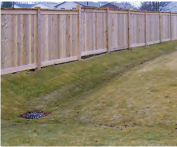
Typical backyard swale with a drain.
